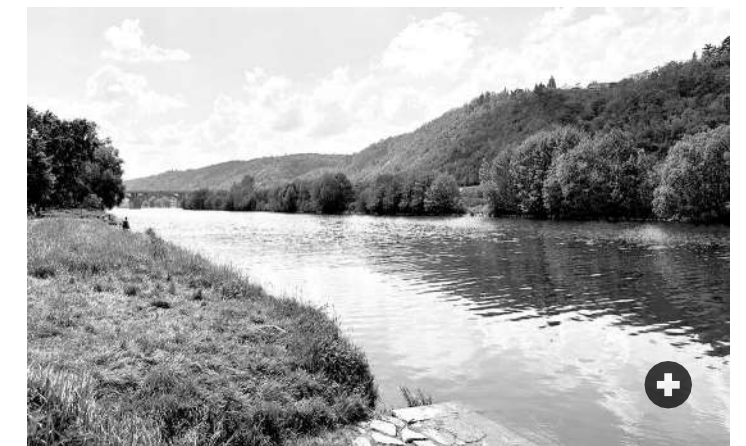
Braník Bridge upstream along the Vitava River
